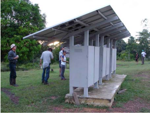
Fig. 5. Sangnilaya Miskito Indian village 2.4 kWp PV battery charging station in the Waspam can charge 24 batteries at a time.
